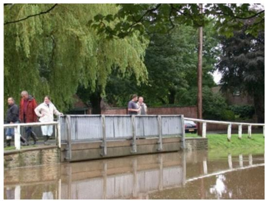
The water is actually on its way down in this picture of the Fullicar Lane bridge. A ditch/channel has been constructed since then in an attempt make a shortcut before water reaches the bridge. The idea is that this should divert some of the water across the road and back into the beck without being held up at the bridge.
